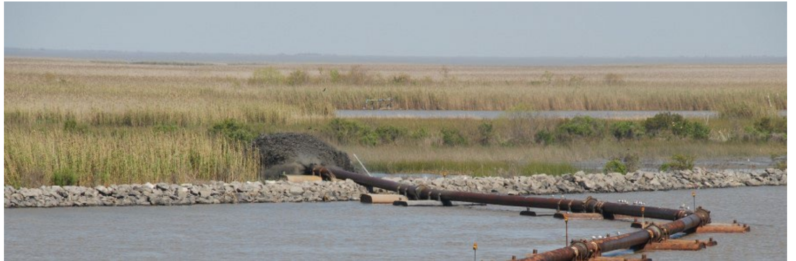
Direct placement of fine-grained dredged material for an engineered marsh (USACE)
